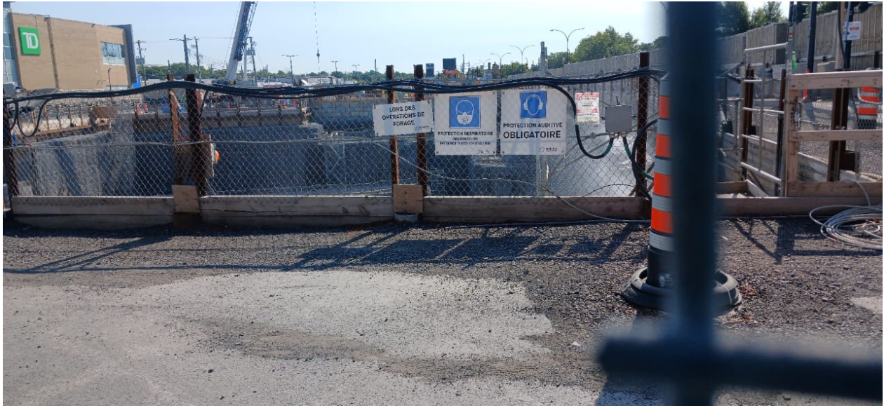
Figure 3 Station Madeleine-Parent en cour de construction (Moussa Touré, 2025).
