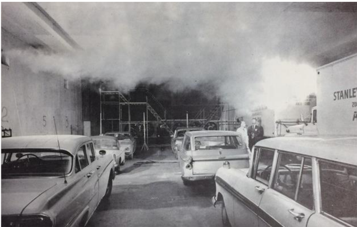
Figure 5.14 Tests de ventilation aux usines de Canadair, 1963
