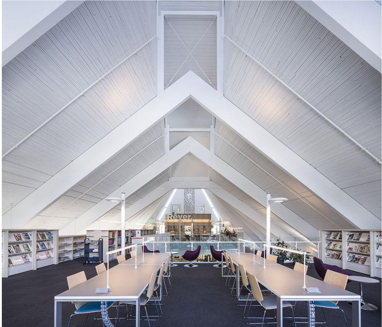
Figure 39. Uniformisation du platelage via un traitement en blanc , INT Design, https://int.design/en/projects/the-monique-corriveau-library/ .
