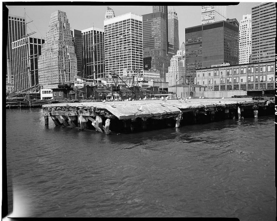
Figure 4.11 Façade arrière du Tin Building et état délabré du quai 17, 1976. « View northwest, detail of the end of pier 18 from the water – South Street Seaport, Piers 17 & 18, South Street into East River at Fulton Street, New York County, NY », HAER NY, 31-NEYO, 145A, Historic American Engineering Record, Library of Congress Prints and Photographs Division, Washington
