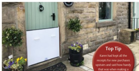
Flood Barrier to basement door and window.
