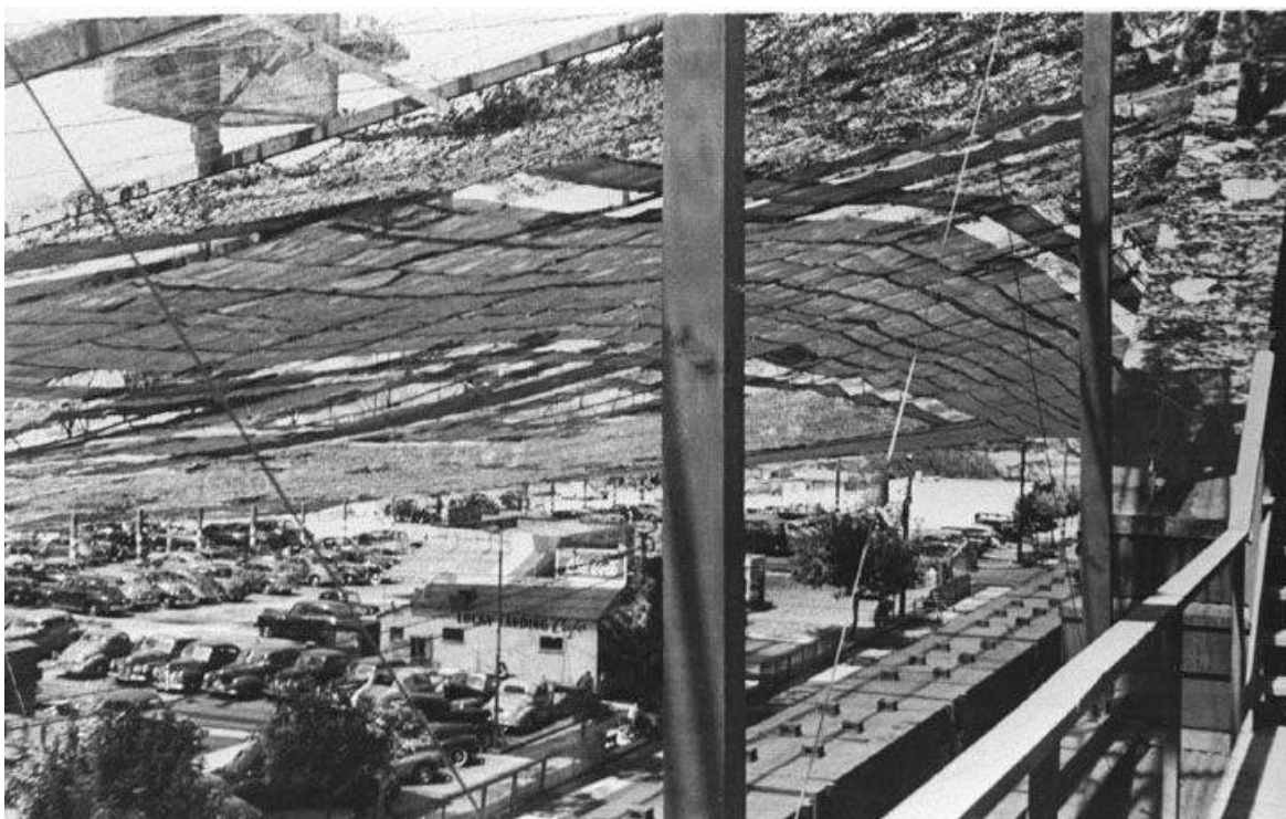
Figure 1.2 Vue sous les filets de camouflage entre 1941 et 1945, View of automobiles parked underneath the camouflage designed by landscape architect Edward Huntsman-Trout to conceal the manufacture of military aircraft at the Douglas Aircraft Company Santa Monica plant during World War II. Santa Monica Public Library archives, https://digital.smpl.org/digital/collection/smarchive/id/3734
