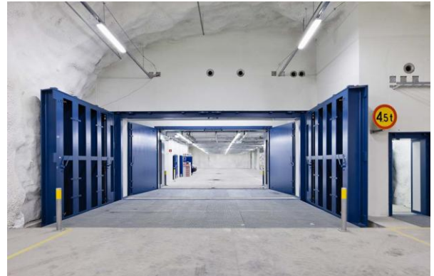
Figure 4.8. Duo de portes de protection , Rockplan, https://www.rockplan.fi/en/services/urban-infrastructure/metro-transportation-and-parking/
