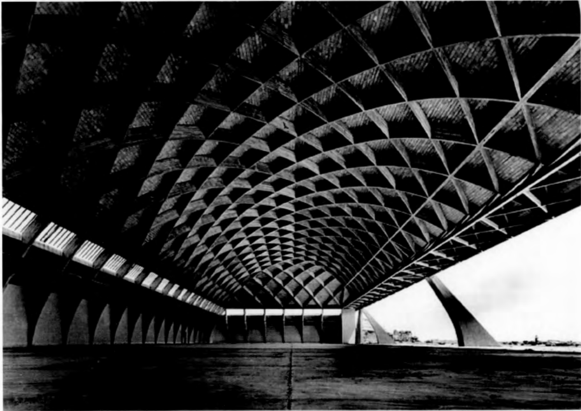
1.13 Pier Luigi Nervi, Orvieto Aircraft Hangar, 1938 (destroyed in 1944). Reinforced concrete structure. Orvieto, Italy. From Tang 2015 , p. 3.
