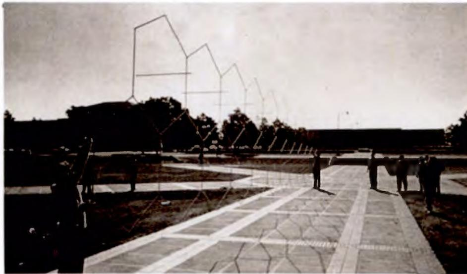
Figure 2-104 - Jeffrey Lindsay (Juillet 1957) 55' shell truss beam, on edge, weighs only 55 lbs. Under load, it revealed some fundamental characteristics of beams which have contributed to more efficient structural design. [Photographie] *Arts and Architecture*
