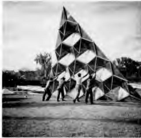
1. Geodesic Pipe Frame (3" o.d. x .063" 6061T6 aluminum alloy) installed over tank. Weight: 1800 lbs. "Shell Truss" panels ready for installation can be seen in the foreground. Components entirely aluminum alloy and stainless steel.
