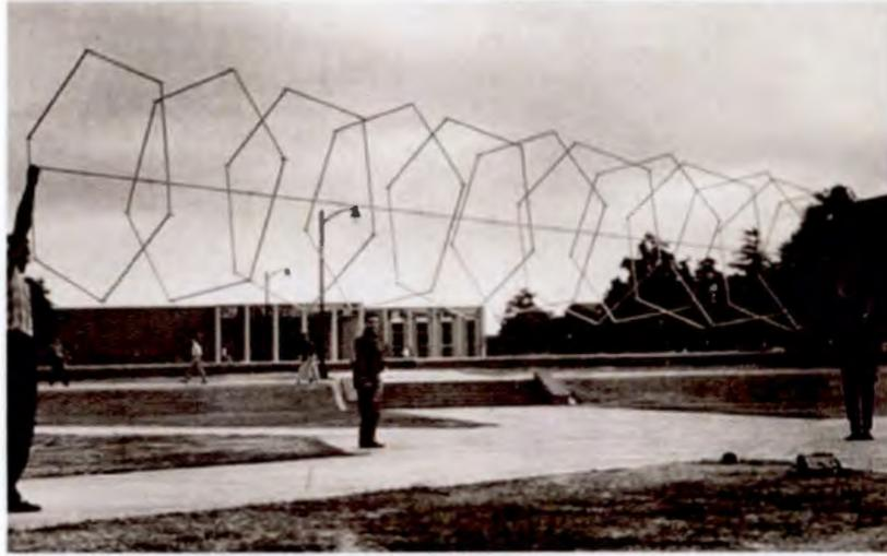
Figure 2-105 - Jeffrey Lindsay (Juillet 1957) *The shell truss tower, horizontal, showing configuration and structural integrity.* [Photographie] Arts and Architecture
