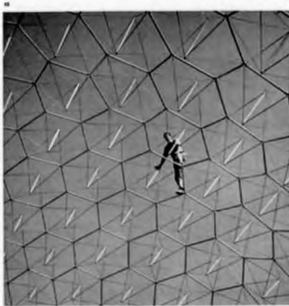
Figure 2-95 – Jeffrey Lindsay (Juillet 1957) Shell truss configuration, a perfect space frame system. Complete separation of tension and compression functions with no more than three members meeting at a point. [Photographie] Arts and Architecture
