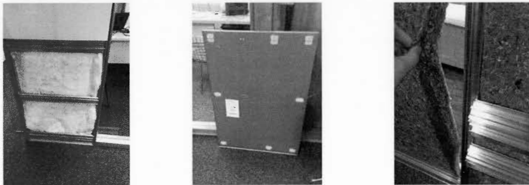
Figure 3.17. This figure shows the basic components of the DIRT partition system, Burovision, Montreal, 2017. Photos by S. Sadraee
