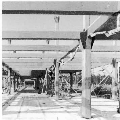
Figure 3.3. This figure shows the columns and beams during the construction, exposed and connected by stand-off steel rod lower chords and bolts. © J. M. Post, XX Architecten.
