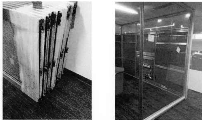
Figure 3.23. This figure shows the prefabricated and preassembled transparent laths, Gaz Métro, Montreal, 2017. Photos by S. Sadraee
