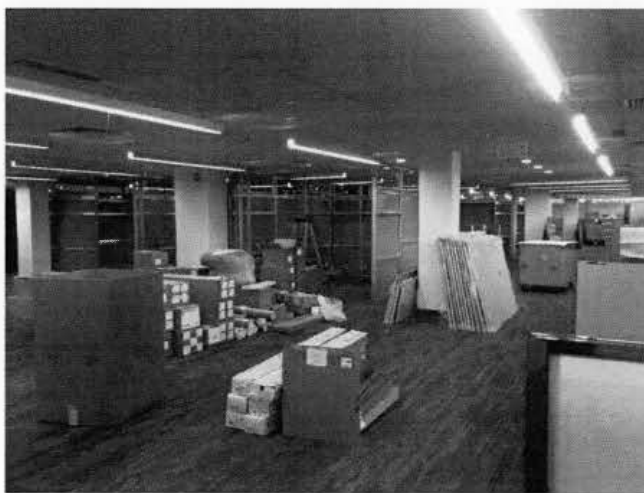
Figure 3.16. This figure shows the DIRTT prefabricated modules ready to be assembled on-site in the Gaz Métro office in Montreal in 2017. Photo by S. Sadraee
