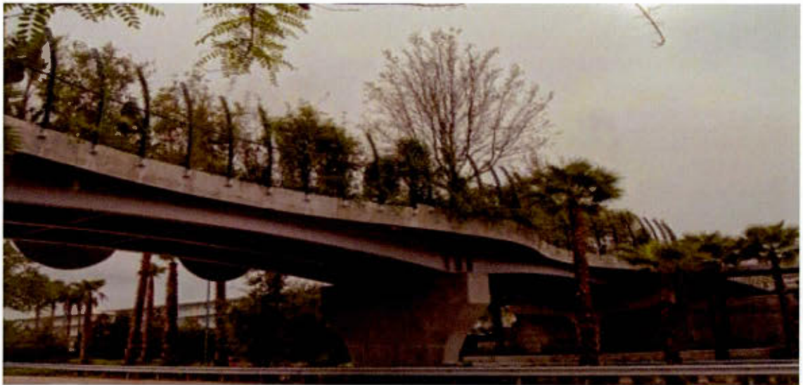
Figure 1.3 : Florida Green Bridge
